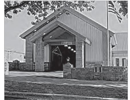
Where newer energy codes require higher levels of insulation, post frame is a particularly good option because its walls and roofs are relatively easy to insulate. Wide column spacing allows for continuous insulation between structural elements, fewer interruptions in insulation material, and less chance of thermal leakage.
